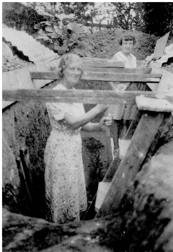
A twelve-year-old girl helping to dig a trench for air raid protection in Kent, 1939. ( D. Rice )
