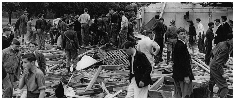
Derek Clark's school, semi-demolished overnight by a doodlebug in 1944.
