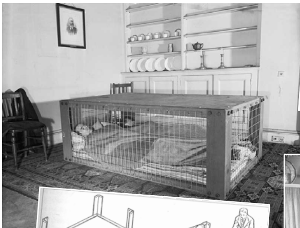
Below: The Morrison shelter was a very strong cage-like shelter inside the home. When not in use, there were many alternative uses for the structure.
