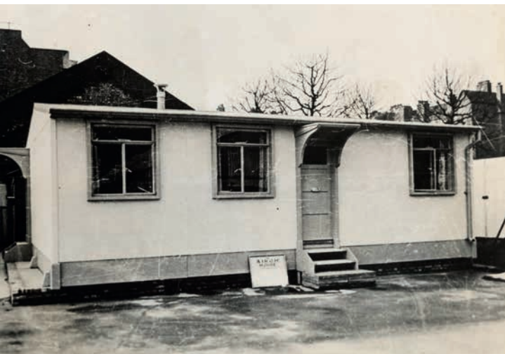
One of the prefabricated houses introduced towards the end of the war in an effort to alleviate a looming housing crisis in Britain's towns and cities. This is an example of the 'Aluminum House' pictured in April 1945. Designed by the Aircraft Industries Research Organization on Housing, it was made in four sections, each complete in itself, which are fastened together a few hours after arrival on site. ( Historic Military Press )
