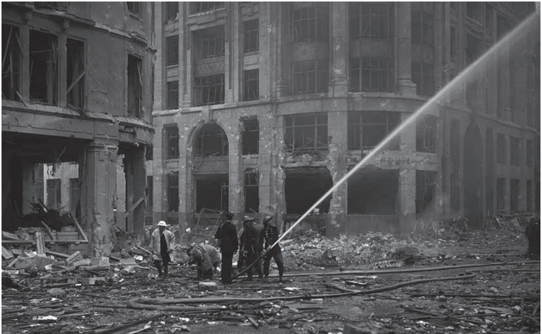
Firemen spray water on damaged buildings, near London Bridge in the City of London, on 9 September 1940. ( Historic Military Press )
