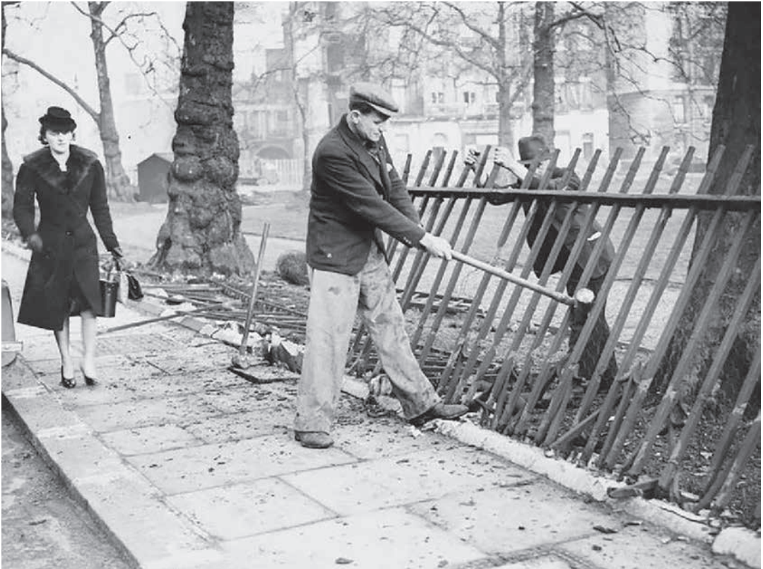
Railings being salvaged for the war effort in Berkeley Square, Mayfair, London, on 3 March 1941. (Public Domain)
