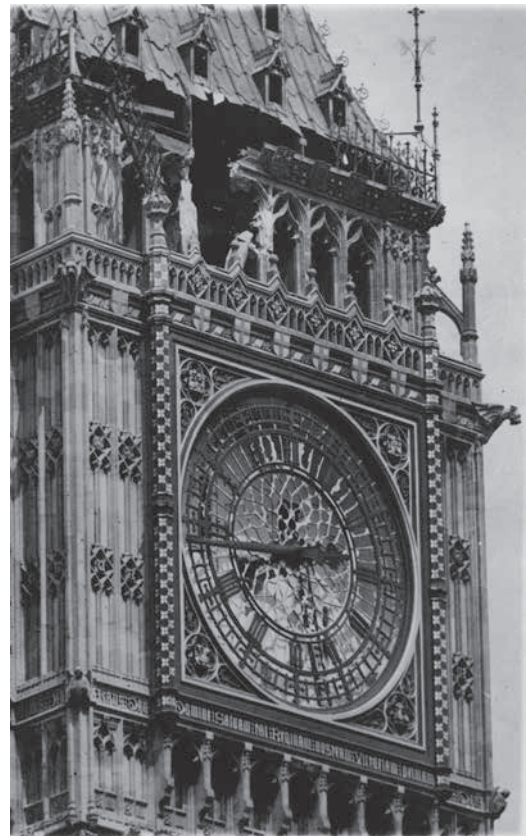
A photograph showing the damage caused when a bomb tore a hole in the stonework of Big Ben during the bombing on 10 May 1941. ( Historic Military Press )
